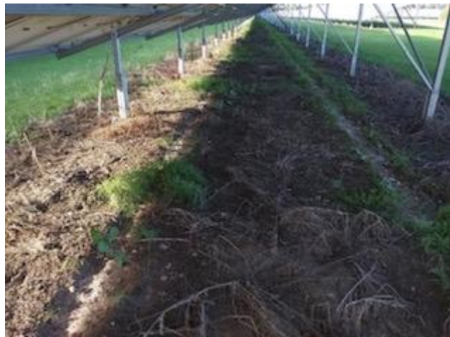
Figure 6 Channels created by panel runoff within 12 months of site operation commencing (Welsh Government (2020) Soil policy evidence programme 2020/21 “The Impact of solar photovoltaic (PV) sites on agricultural soils and land”)
